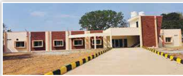
HAL has constructed Sports Hostel at Kolar
