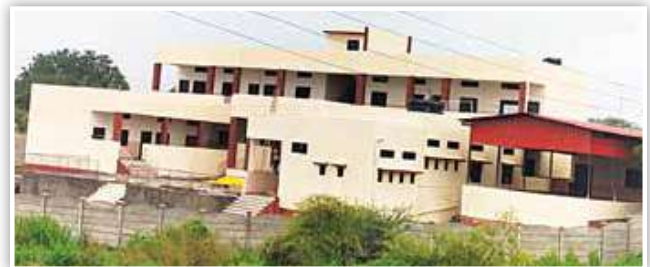
HAL has constructed Zilla Parishad School at Nasik
