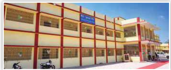
HAL has constructed Health Care & Rehabilitation Centre for Homeless & Mentally Challenged Women at Koraput
